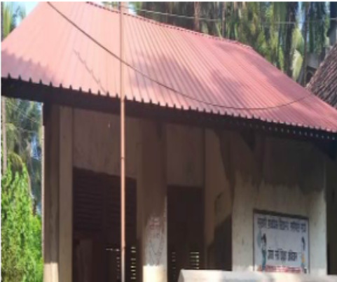
Polling Station Building Front View
