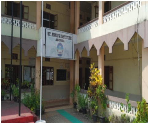
Polling Station Building Front View
