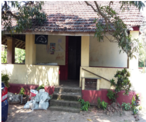
Polling Station Front View
