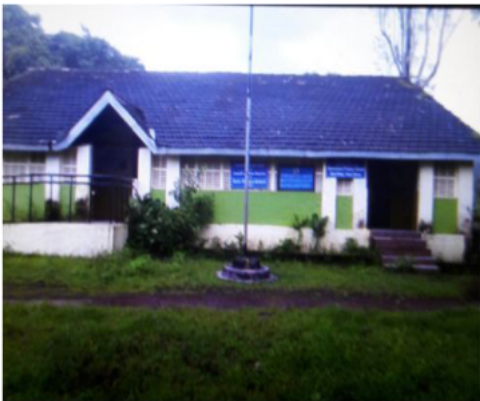
Polling Station Building Front View
