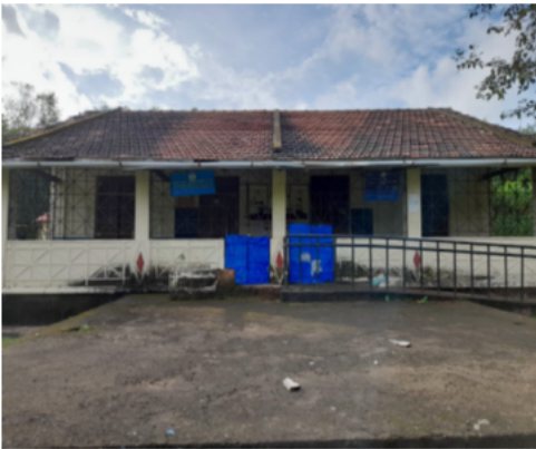
Polling Station Building Front View
