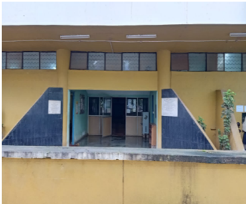
Polling Station Building Front View
