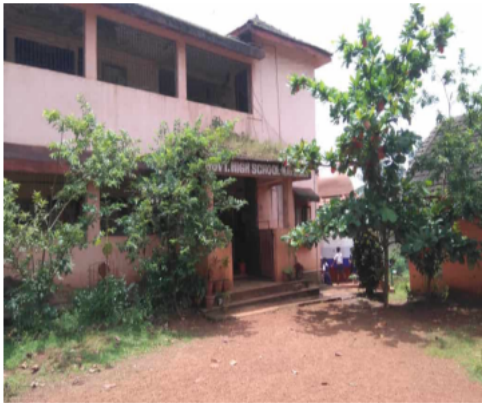
Polling Station Building Front View
