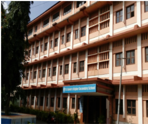
Polling Station Building Front View
