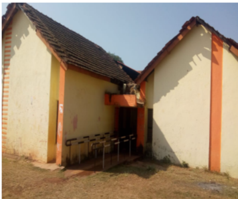
Polling Station Building Front View
