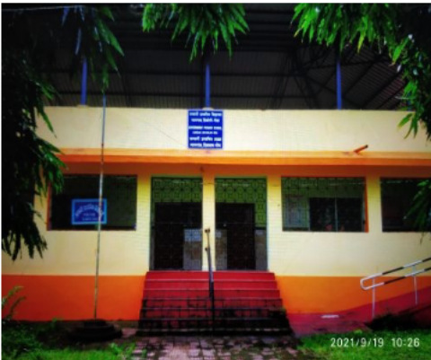
Polling Station Building Front View
